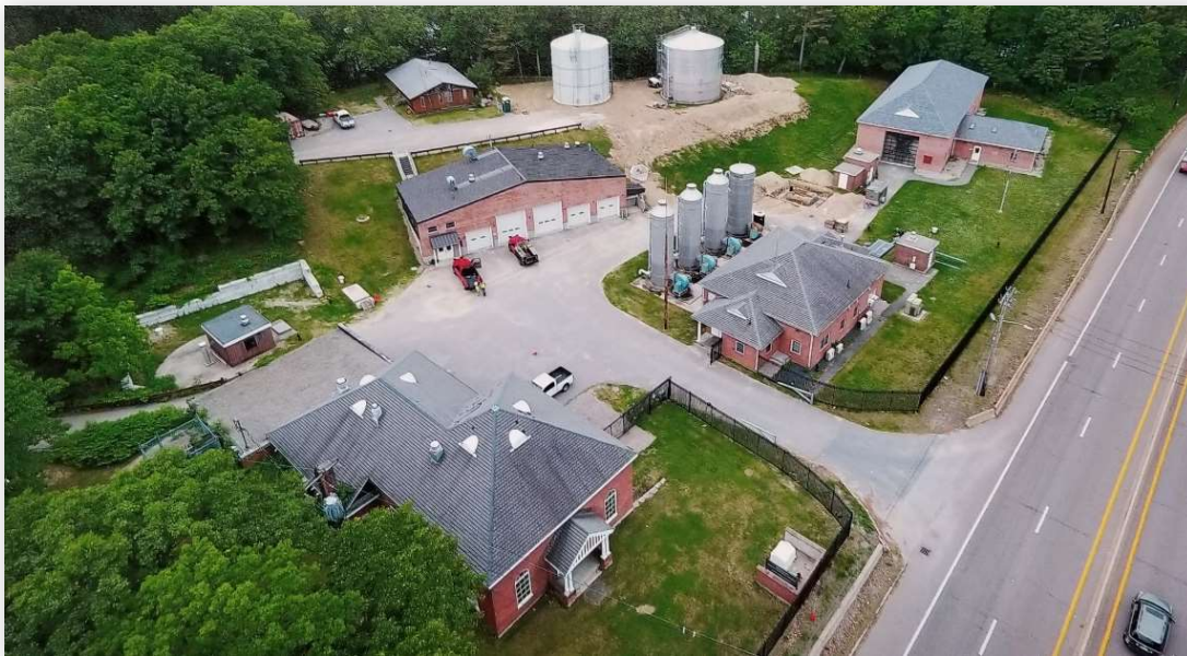
Figure 8. Natick Water Treatment Plant
